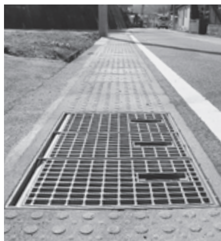
▶ 間沢地区内の流雪溝
